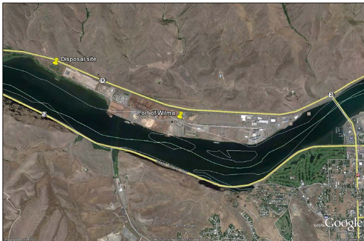
Figure L-22. Port of Wilma Site
