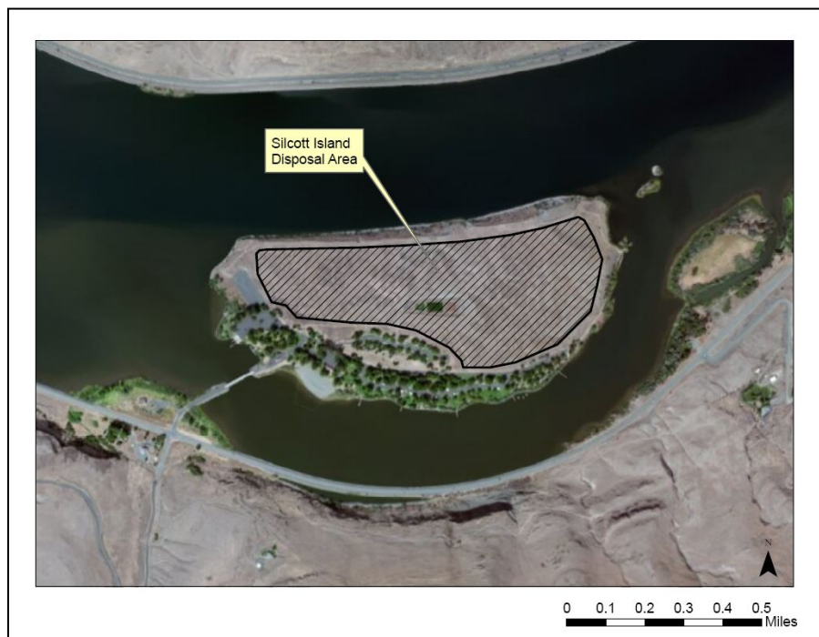
Figure L-20. Silcott Island Site
